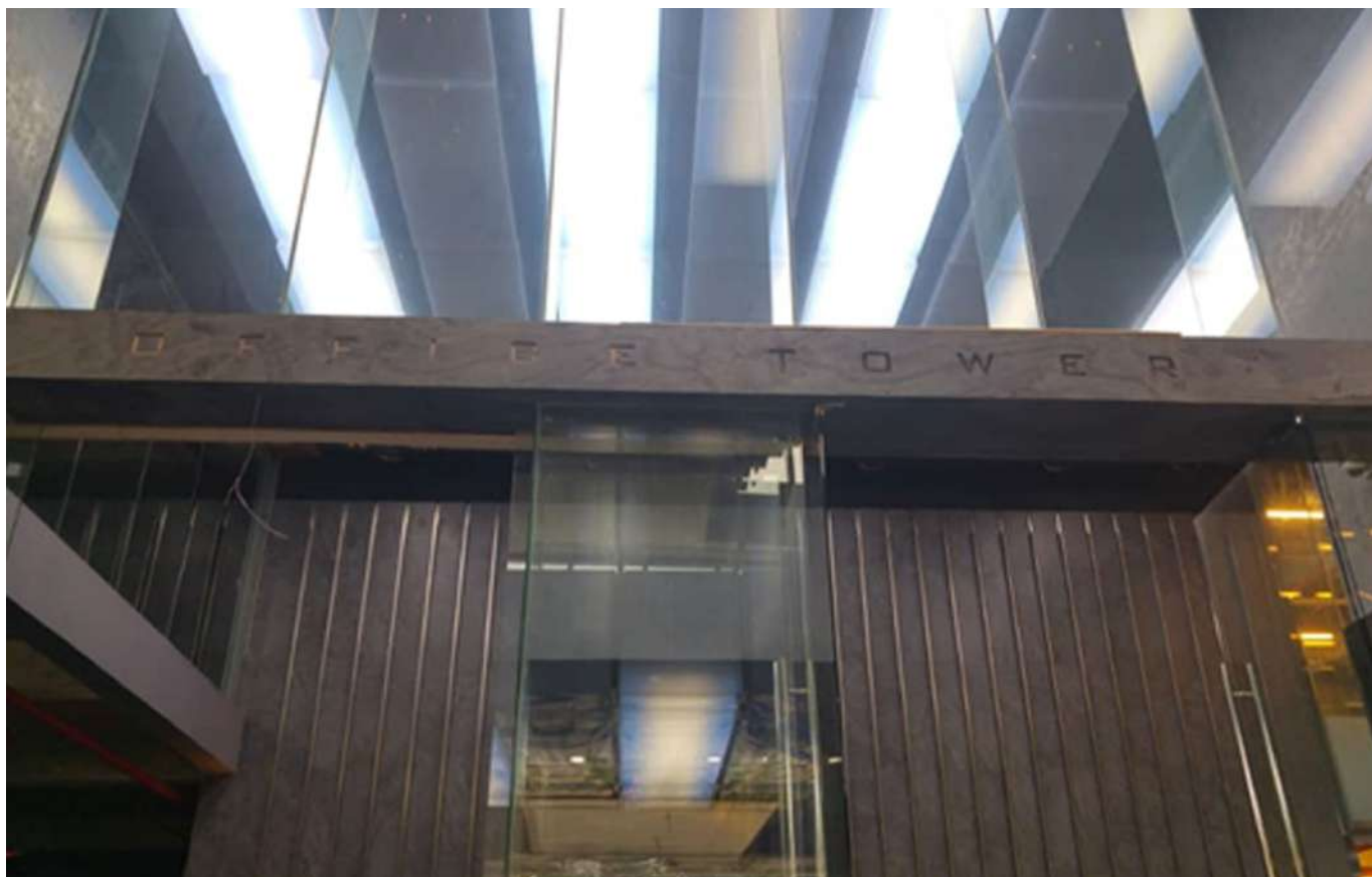
OFFICE TOWER J/B, SUBANG MALAYSIA, DEKOR STEEL BLACK
